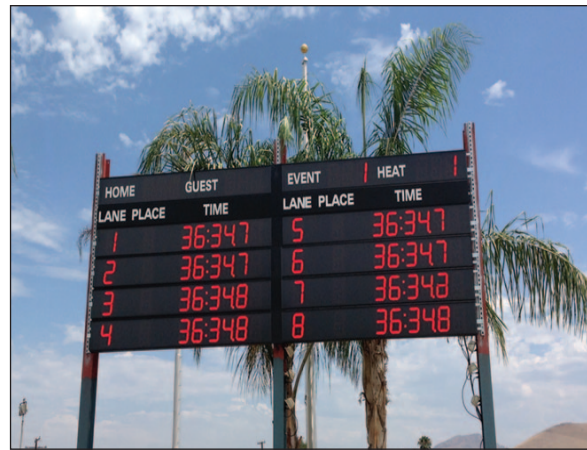
Repaired Timing System at the WHS Pool
