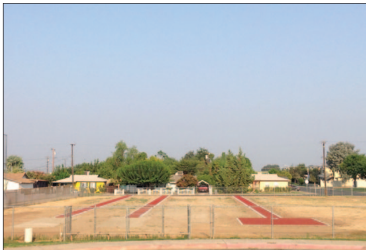
Completion of Track and Field at the New WHS Stadium
