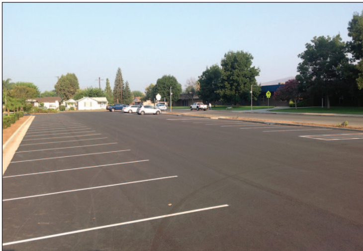
Repaved Parking Lot at the Memorial Building across from WHS
